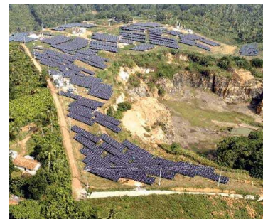
Panasian Power is a pioneering supplier of renewable energy in Sri Lanka.
